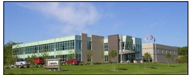
MEPPI Headquarters located in Warrendale, PA
