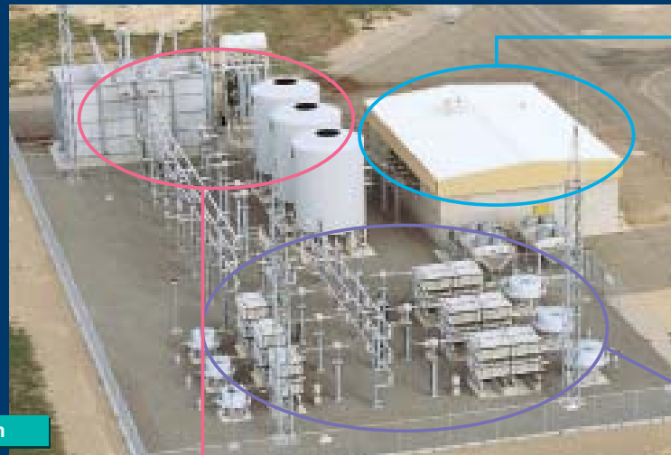
4 SVC Transformer 5 TCR Reactor
